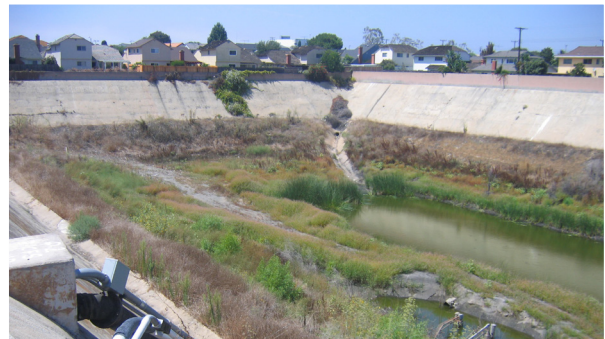
Torrance Detention Basin. Enhancement of detention basins in the Dominguez Channel watershed could improve water quality, create habitat, and provide passive recreation opportunities.
