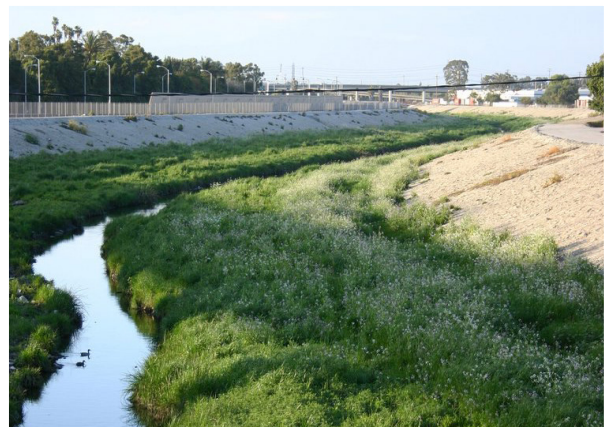
Compton Creek. Restoration of the natural bottom section of Compton Creek could improve water quality, facilitate recharge, and restore habitat.
